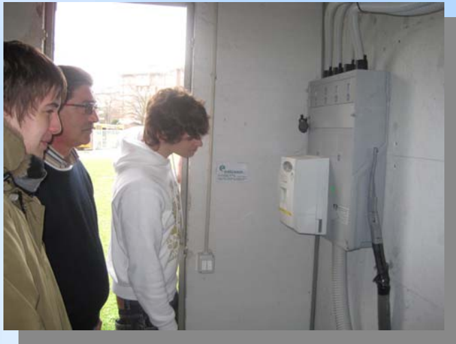
daily check of all electrical consumption
